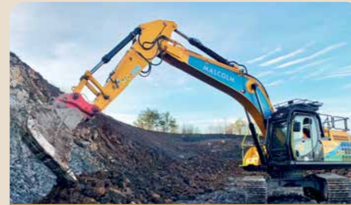
JCB JS300 TRACKED EXCAVATOR
