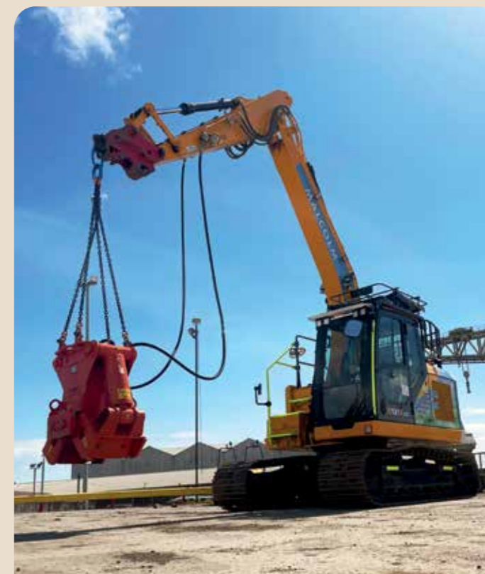
JCB JS131 TRACKED EXCAVATOR WITH CROPPER
