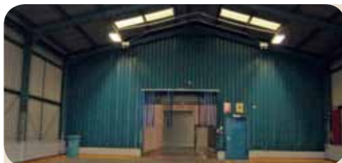
Malcolm Logistics' G Shed at Burnbrae Road.
