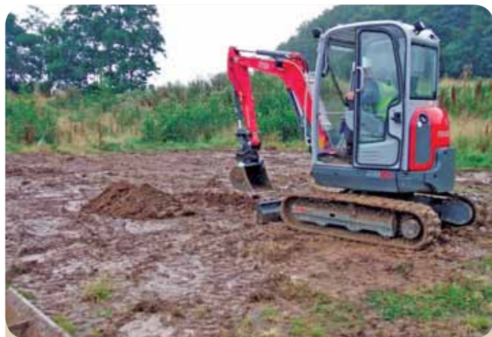
Operating the machine is Nicky Rea.
